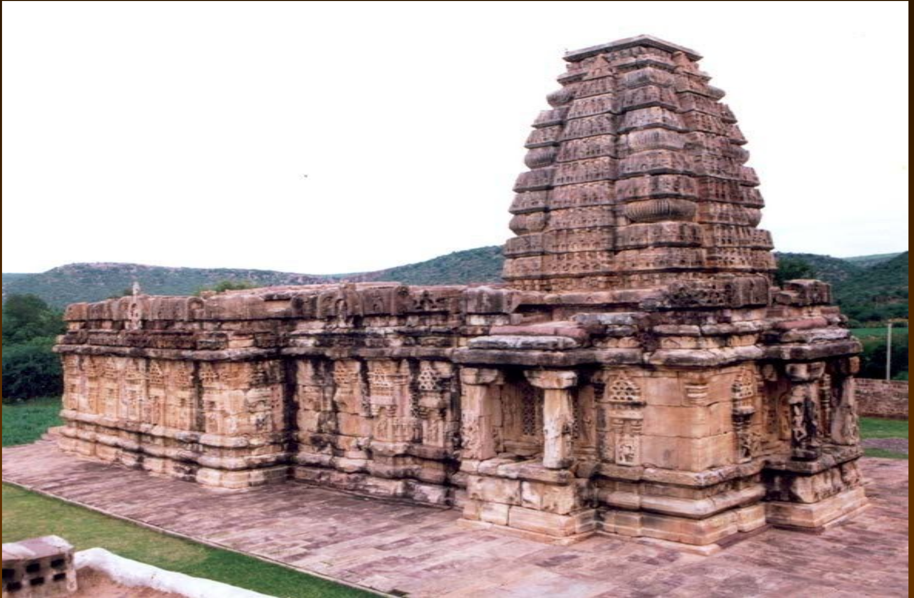
Papanatha temple, Pattadakal, 750 AD, northern Rekha Nagara with some southern vimana components, Mixed idiom. Note eg. hara , kudyastambha components
