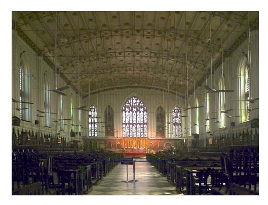
"The roof is unusual. It is a shallow curve spanned by iron trusses adorned with Gothic tracery," explains Davies: "when built, it was one of the largest spans in existence"
