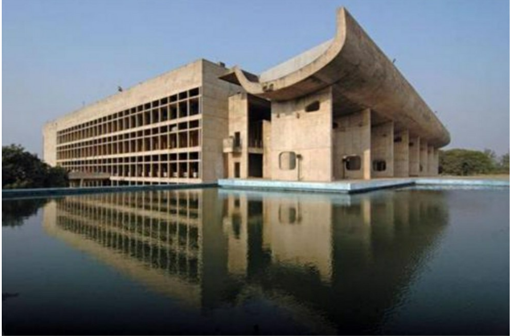
Capitol complex, Chandigarh
